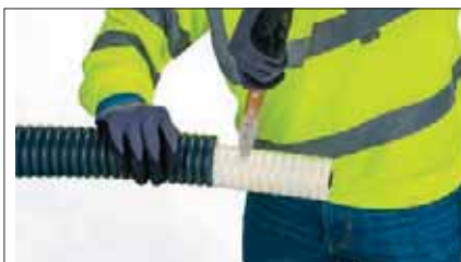
5 Cut back/remove the insulation along the length (x, y, z). Caution: Do not damage the medium pipe.
