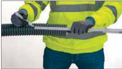
1 Mark the sheath the distance (x, y, z) +1 cm from the end of the pipe.
