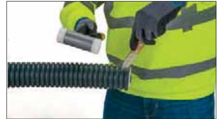
3 Cut the sheath open lengthways. Do not insert the blade more than 5 mm deep. Caution: Do not damage the medium pipe.
