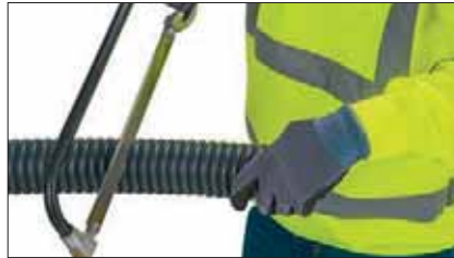
2 Cut through the sheath with a saw.
