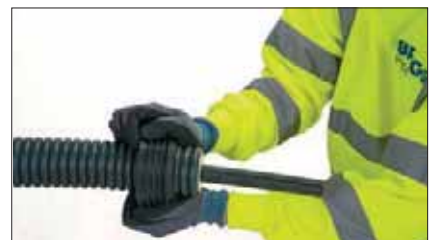
6 Install the wall sealing ring.
