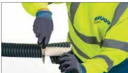
4 Peel off the sheath.
