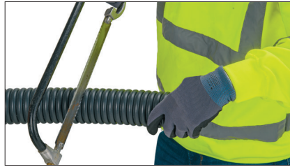
2 Cut through the sheath with a saw.
