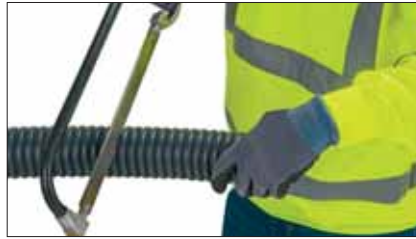
2 Cut through the sheath with a saw.
