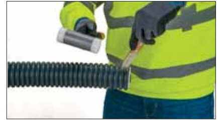
3 Cut the sheath open lengthways. Do not insert the blade more than 5 mm deep.
