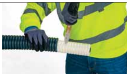
5 Cut back/remove the insulation along the length (x, y, z).
