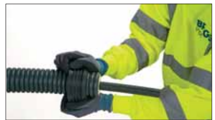
6 Install the wall sealing ring.
