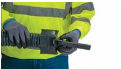
7 Carefully shrink the pipe end cap in line with the enclosed Raychem DHEC installation instructions.
