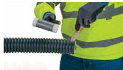
3 Cut the sheath open lengthways. Do not insert the blade more than 5 mm deep. Caution: Do not damage the medium pipe.
