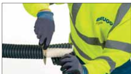
4 Peel off the sheath.
