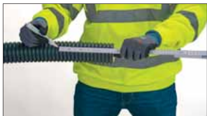
1 Mark the sheath the distance (x, y, z) +1 cm from the end of the pipe.
