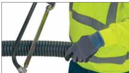
2 Cut through the sheath with a saw.
