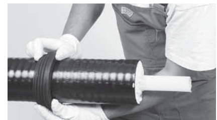
6 Install the wall sealing ring.
