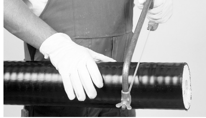
2 Cut the casing pipe with saw.
