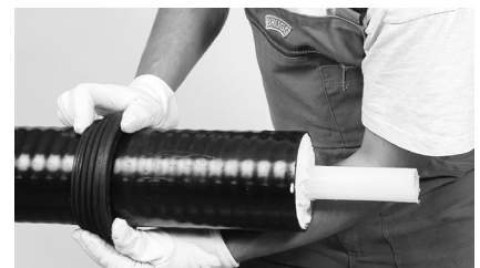
6 Install the wall sealing ring.
