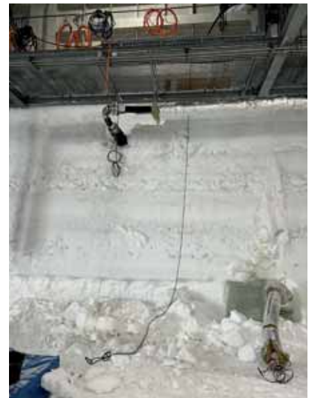
Old and new pipe.
