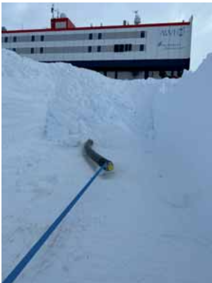
Holding the pipe in the centre of the trench.
