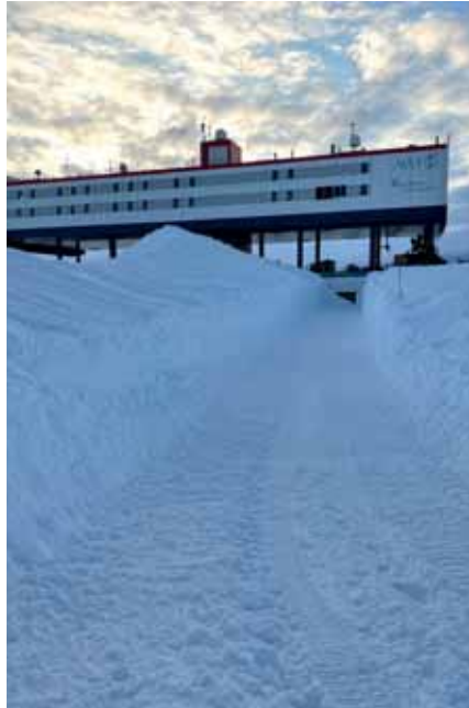
Trench with gradient is finished, length approx. 50 m.
