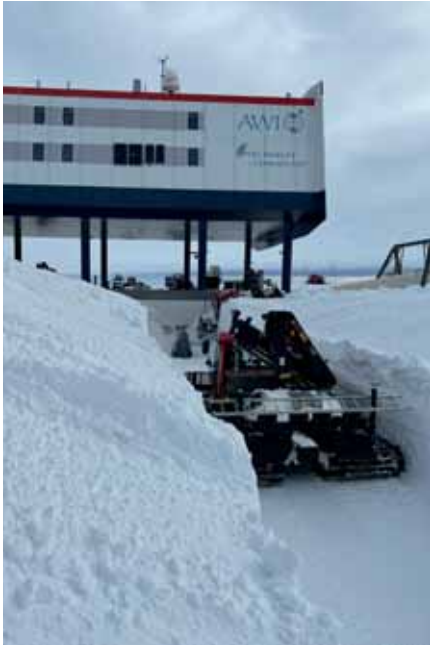
Trench through east hill.
