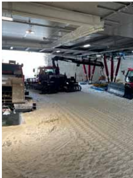
Rotzler winch pulls pipe from drum.
